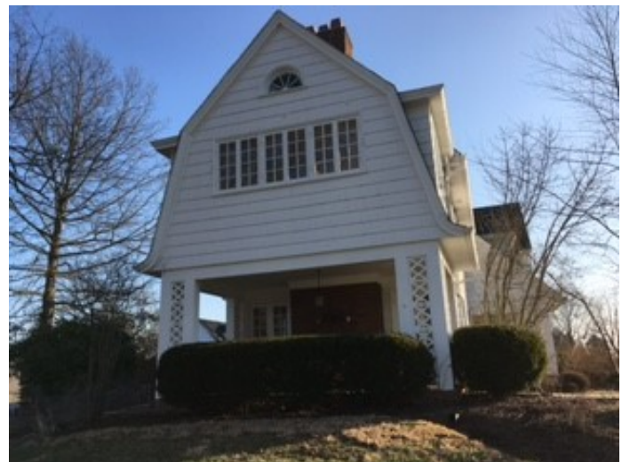
West Side façade
