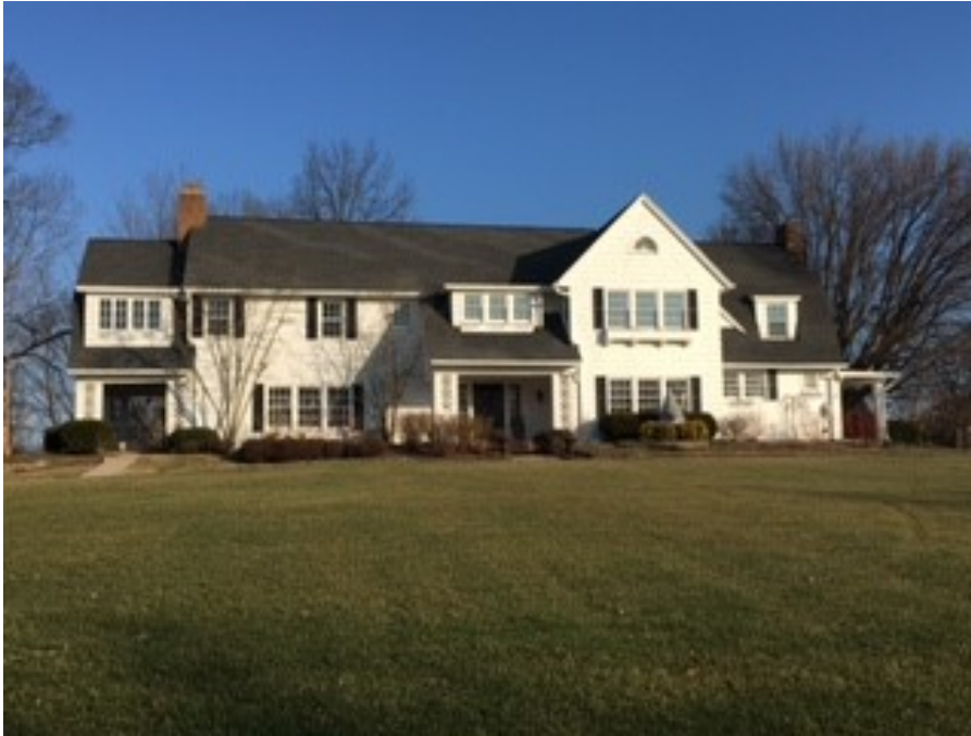
South (main) façade
