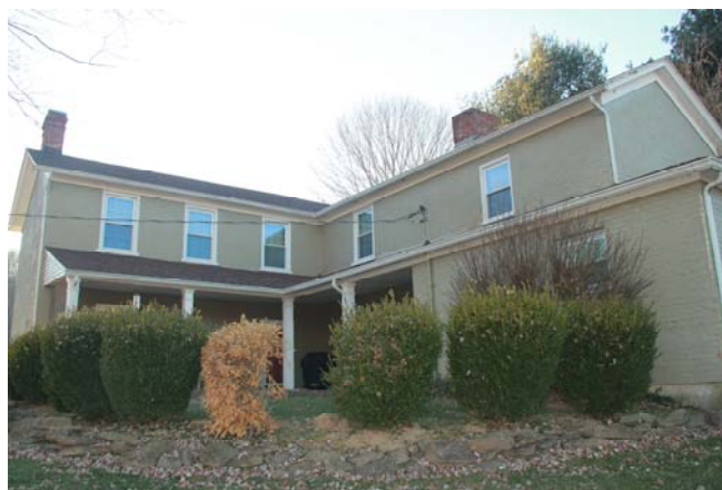
Back side (on left) and east side of ell (at right)
