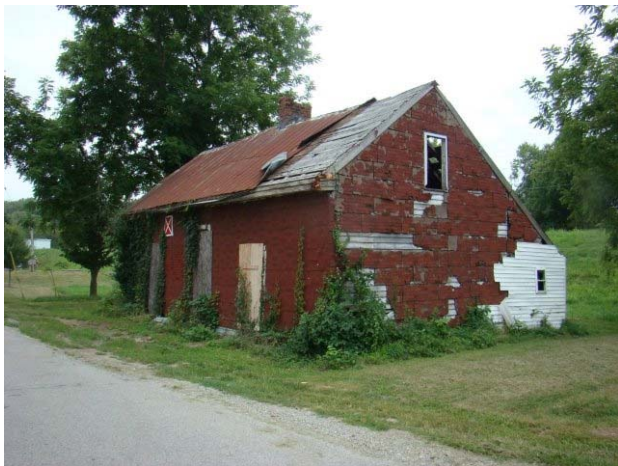
North (front) and west side
