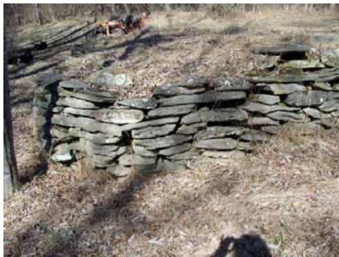
Photo #2 East façade of winery, camera facing west
