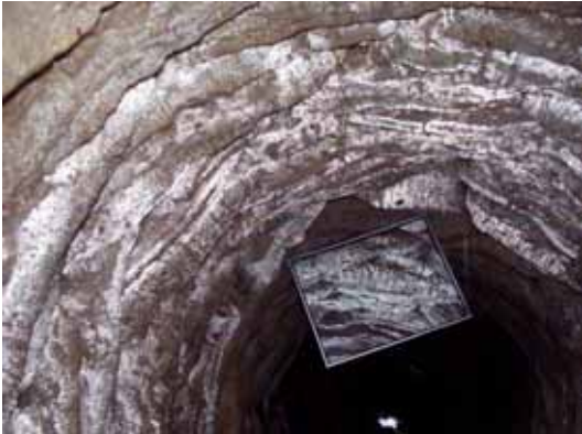
Photo #20 Domed corbelled well
